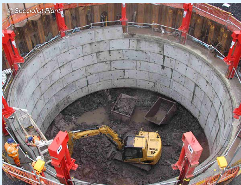
Graphic 3–11 Example of tunnel shaft construction
